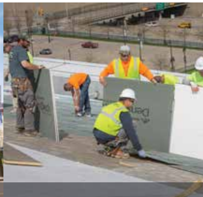
Repair and Replace
