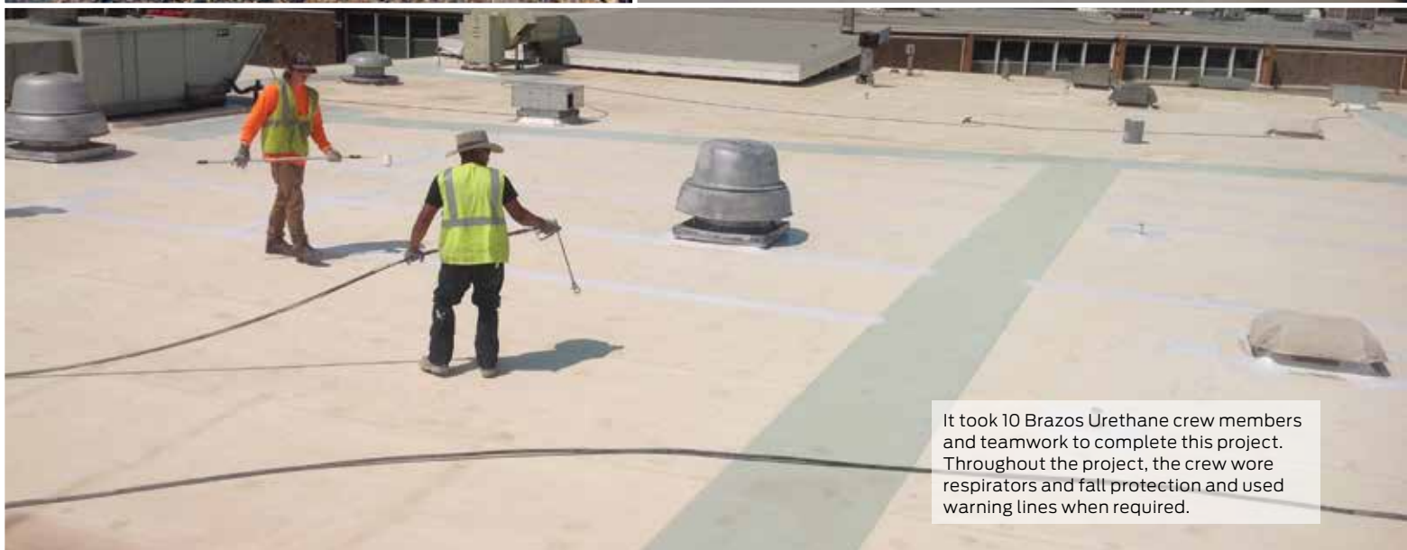
The Brazos Urethane team used two other teams to kick off this approximately 134,700-square-foot (12,514.0 m 2 ) project: A cleaning division washed and vacuumed the poor roofs and another crew surveyed the roof for waterlogged foam.
