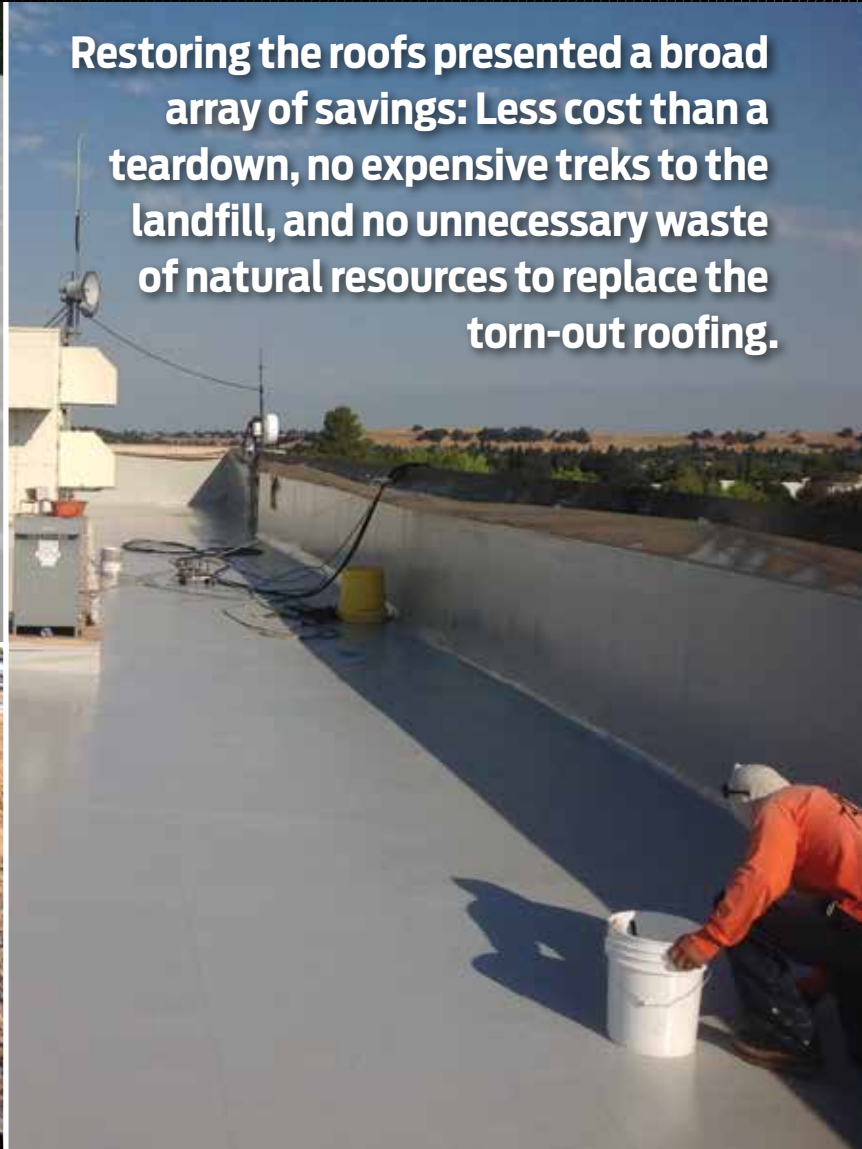
The Brazos Urethane team used two other teams to kick off this approximately 134,700-square-foot (12,514.0 m 2 ) project: A cleaning division washed and vacuumed the poor roofs and another crew surveyed the roof for waterlogged foam.
