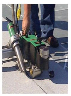
Leister, a leading manufacturer of heat-welding equipment, has developed the Bitumat B2 heat seaming unit for use in the hot air welding of modified bitumen membranes.
