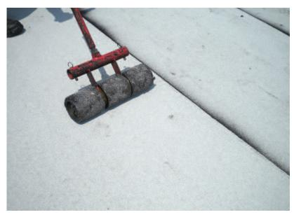
Tremco requires all cold applied POWERply top membranes to be fully rolled into the adhesive immediately after application. A 35 to 75 lb. (16-34 kg) weighted roller improves the contact of the back of the POWERply membrane with the adhesives, to minimize the potential for voids within the roof membrane system.
