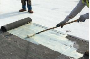
while adhesive is wet. If air pockets are noticed use the roller across the roll to work the air pockets out.
