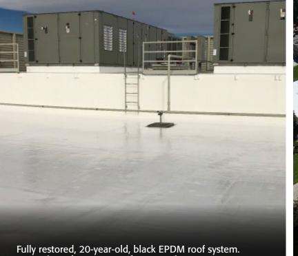
Fully restored, 20-year-old, black EPDM roof system. Approximately 44.4 tons of construction waste was diverted from entering the landfill.
