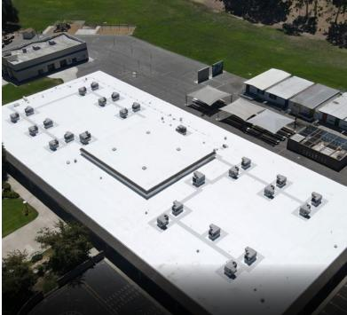
New 42,000-plus square foot single-ply roofing project offers excellent fire rating, and meets ENERGY STAR Roofing Program guidelines.
