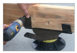
4. Fold Joist Top flaps up to meet the joist. Mechanically fasten flaps to joist with #8 deck the joist has been secured to screws.
