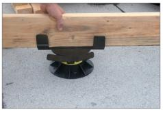
3. Place joist (2x or 4x) on top of the Bison Joist Top.
