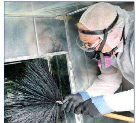
Once the section is under negative pressure, the cleaning can commence. We utilize a variety of tools depending on the physical size and type of duct being serviced. Most often it's a combination of compressed air with a reverse flow nozzle and a Rotobrush application. Each section is worked towards the negative air machine, pushing dust and debris into the immense HEPA vacuum.
